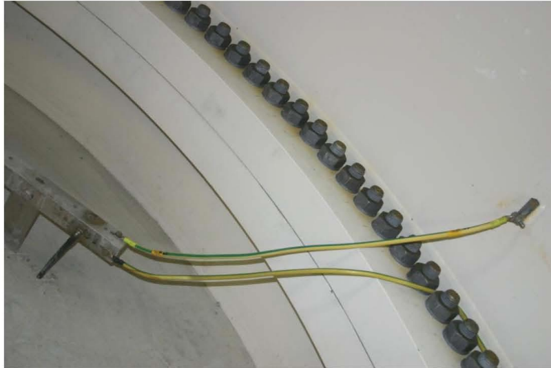
Figure 2-8: Connection between tower and main bonding bar
